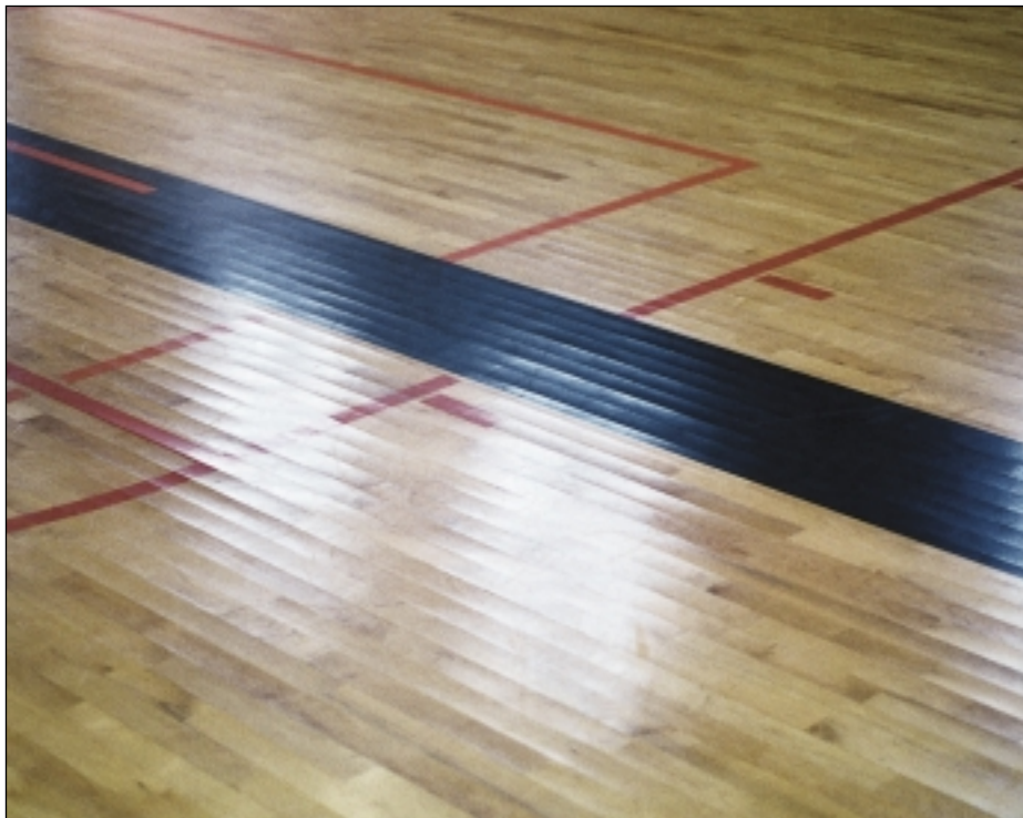
Excessive moisture in the interior environment or from beneath the floor can cause wood flooring to take on moisture. The result can be a "cupped" floor. For more on cupping, see page 19.
